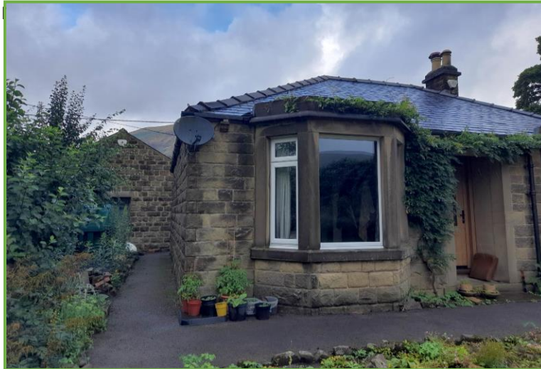
Photo 1: View of Broadlee bungalow and view of western aspect of proposed extension
