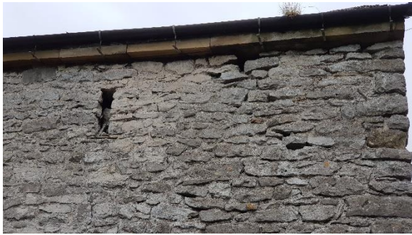
3 - East elevation holes in stonework
