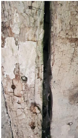
9 - Ground floor - Gap at door lintel
