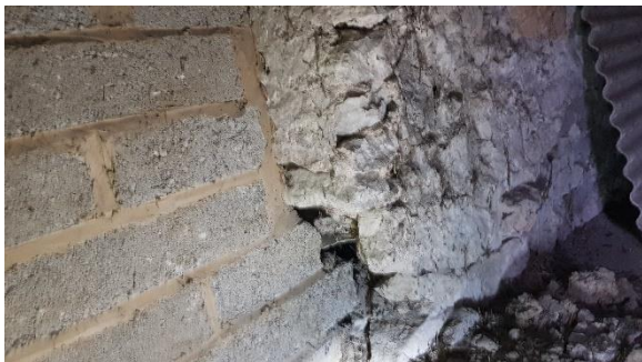
11 - First floor - gap at cement block wall
