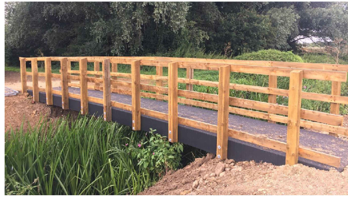
Resin infused FRP (Fibre Reinforced Polymer) bridge as supplied by Lifespan Structures Ltd.
