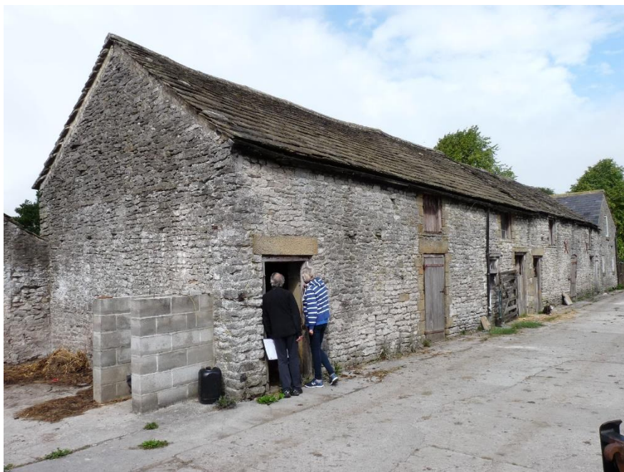
Fig.7: south gable and east elevation from the south-east
