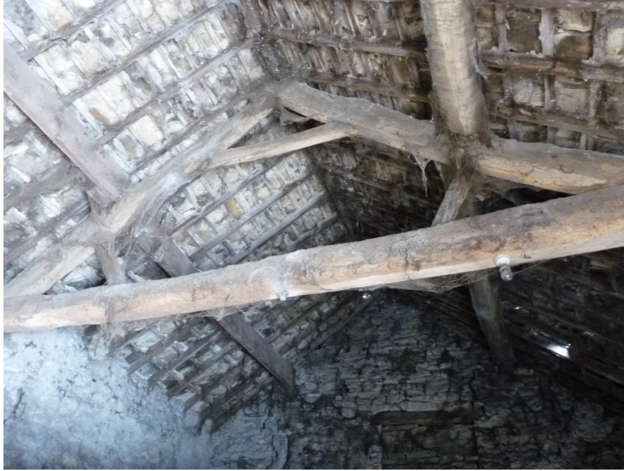
Fig. 16: roof truss in two south bays, from the north.
