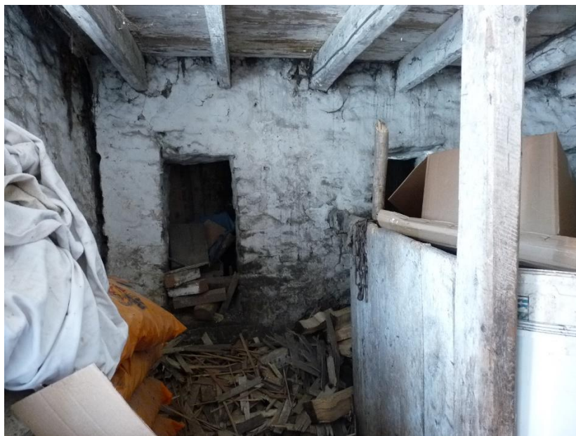
Fig.13: north cow house with timber boskins and feed holes, from the north
