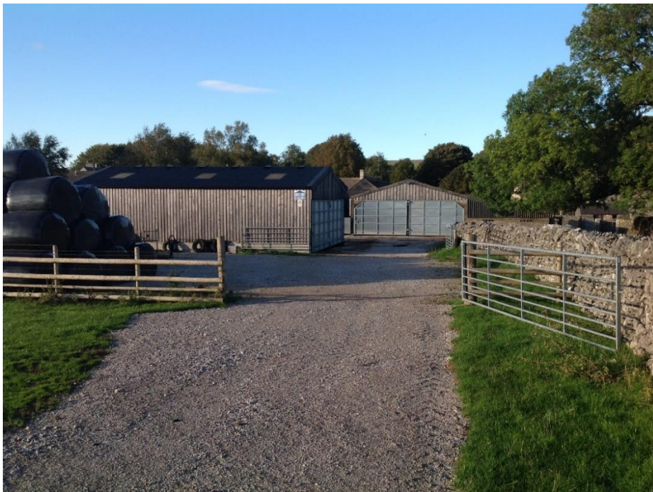
Fig.27: the farmstead from the south, with recent sheds screening views of the older buildings (photo: Robert Hall)
