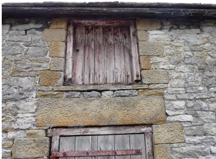
Fig.29: shutter above doorway, south end of main range (east elevation)
