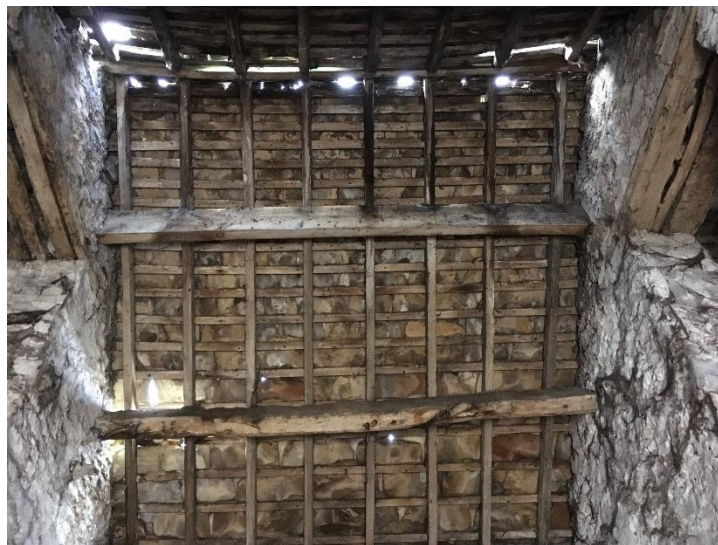
Fig.28: typical roof - centre bay of north shippon
