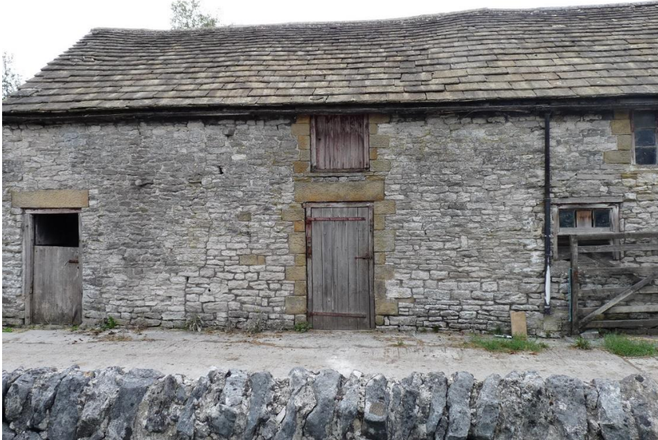
Fig.9: south part of linear range, from east
