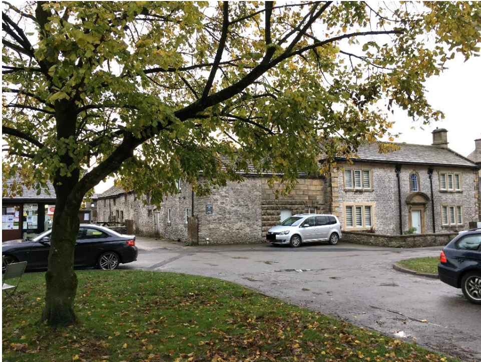
Fig.22: view of the farmhouse and farm buildings from the green
