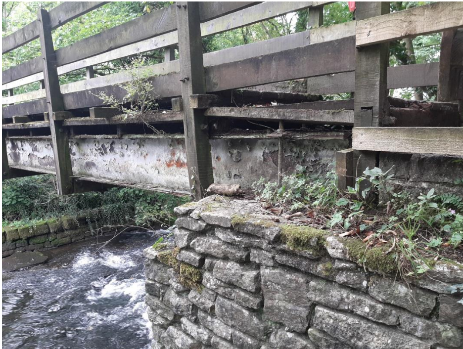
View at Western Abutment showing deck build-up
