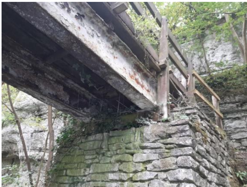
Recess at top of Northern face of abutment
