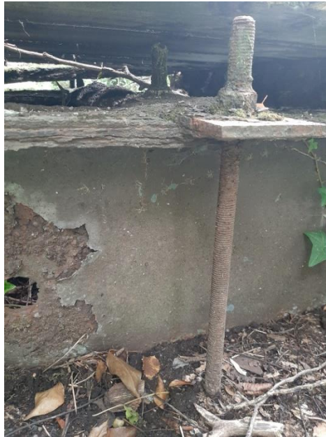
Bridge beam support fixing – Western Abutment, southern side
