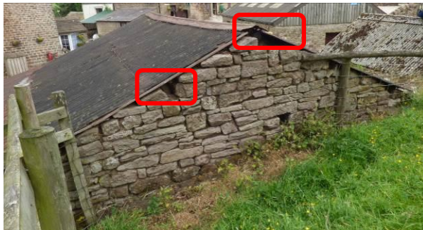
Photograph 15. Example large and open gap beneath the metal roof sheeting of B2b.
