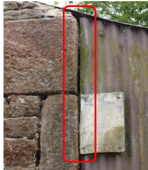
Photograph 18. Stepped crack within the interior eastern stone wall of B2c.
