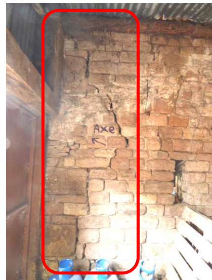
Photograph 18. Stepped crack within the interior eastern stone wall of B2c.
