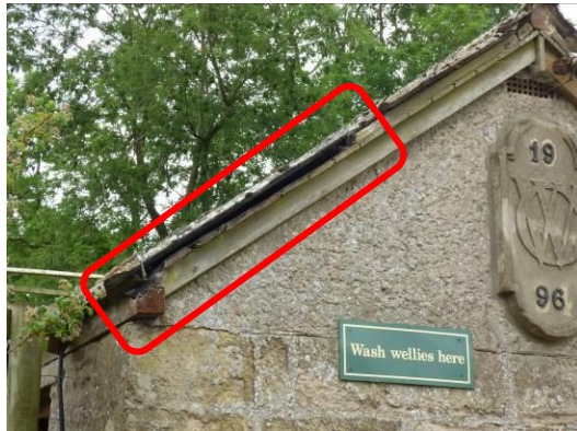
Photograph 11. B2a; location of large open cavity.
