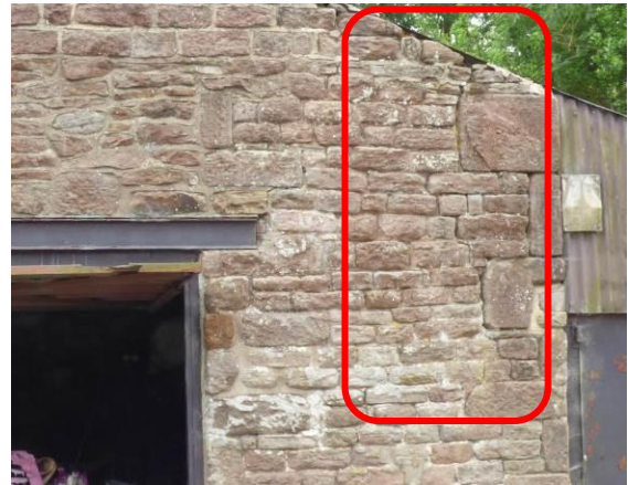
Photograph 16. Vertical gap between B2b and B2c
