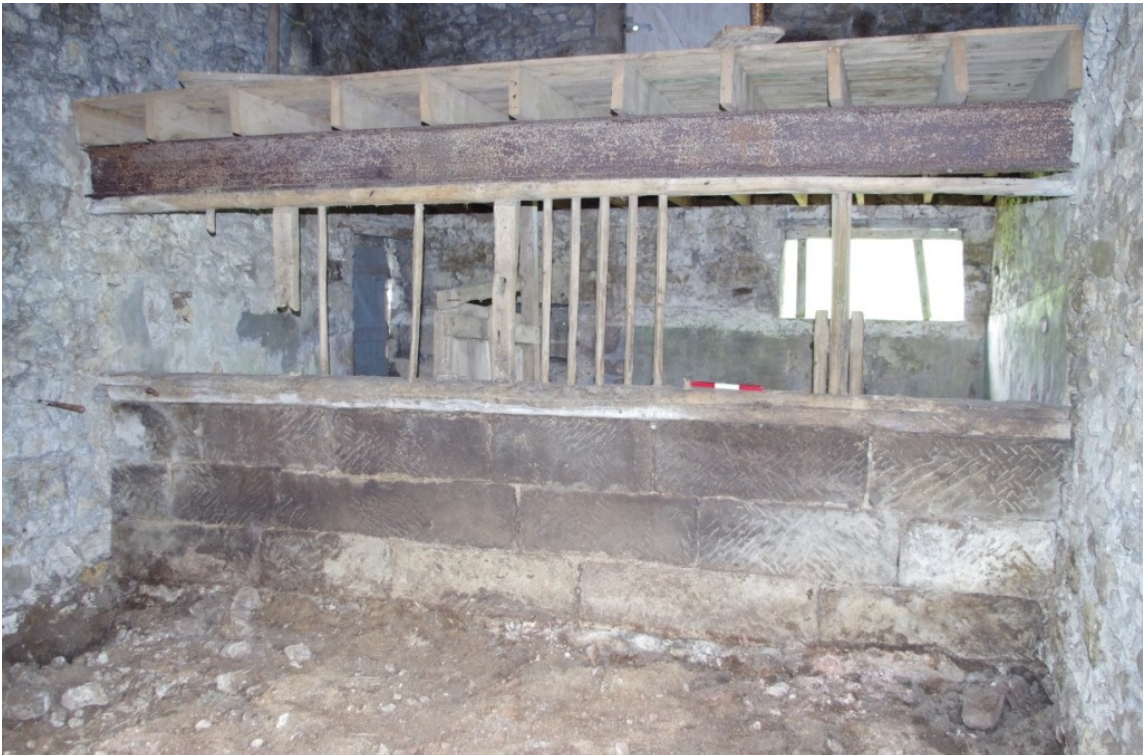
Figure 15 Gritstone Cross Wall & Timber Staves.
