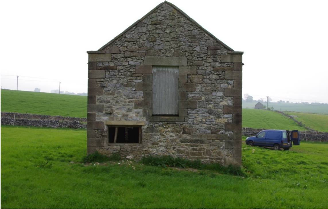
Figure 10 West Facing Gable.
