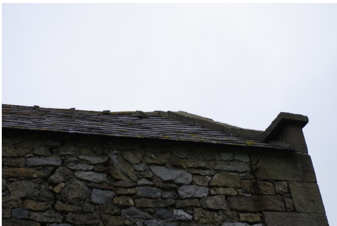
Figure 13 Gable Parapet & Kneelers.
