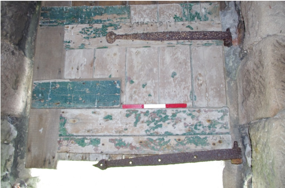
Figure 17 (2) Early Strap Hinges Including 16th Century “Style” Round Headed Hinge (Top).
