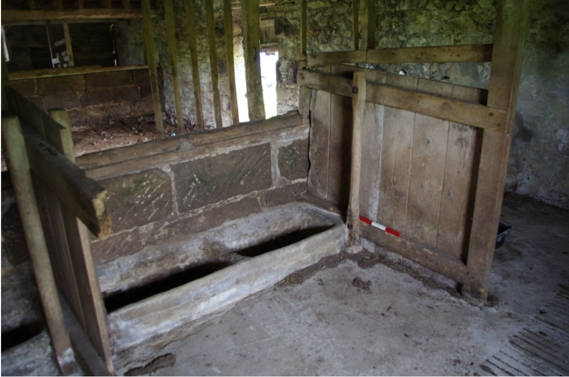
Figure 14 (1) Stalls & Original Tether Bar.
