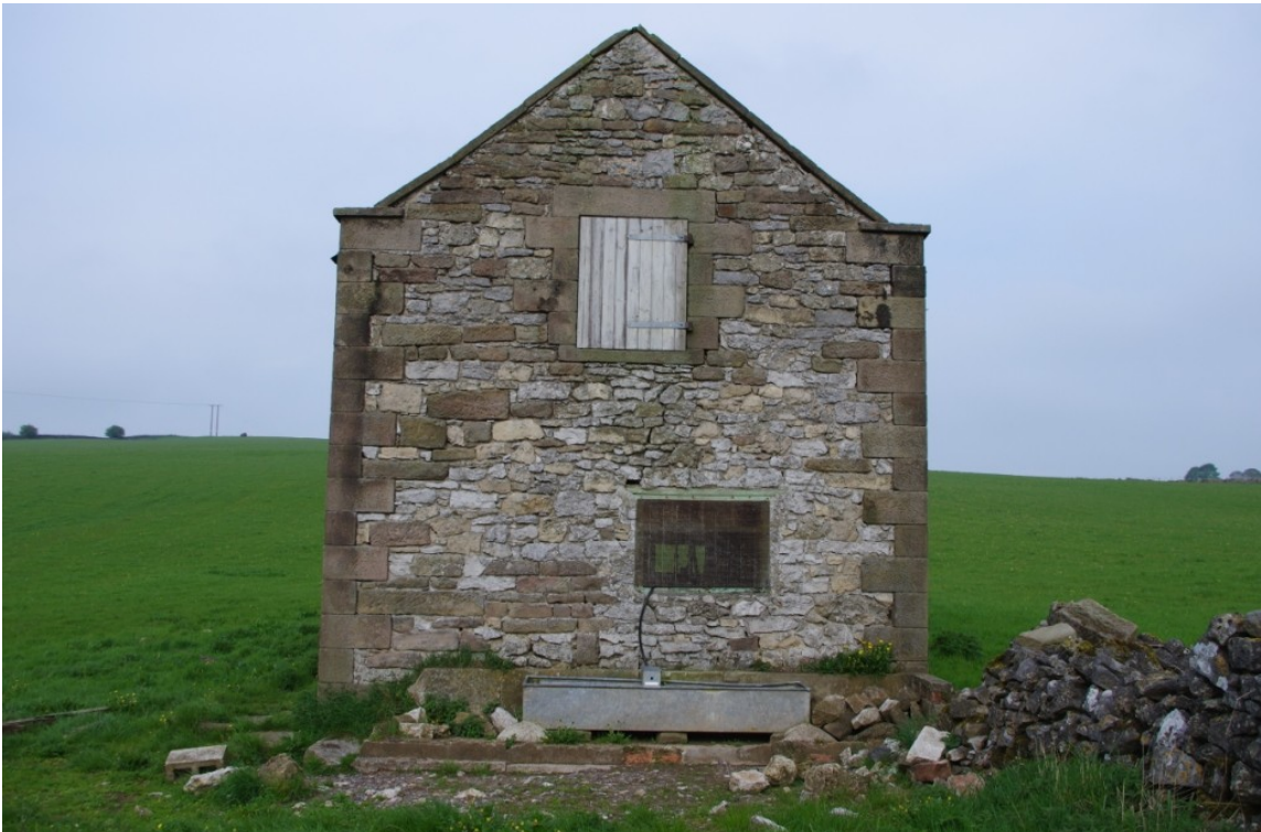
Figure 11 East Facing Gable.
