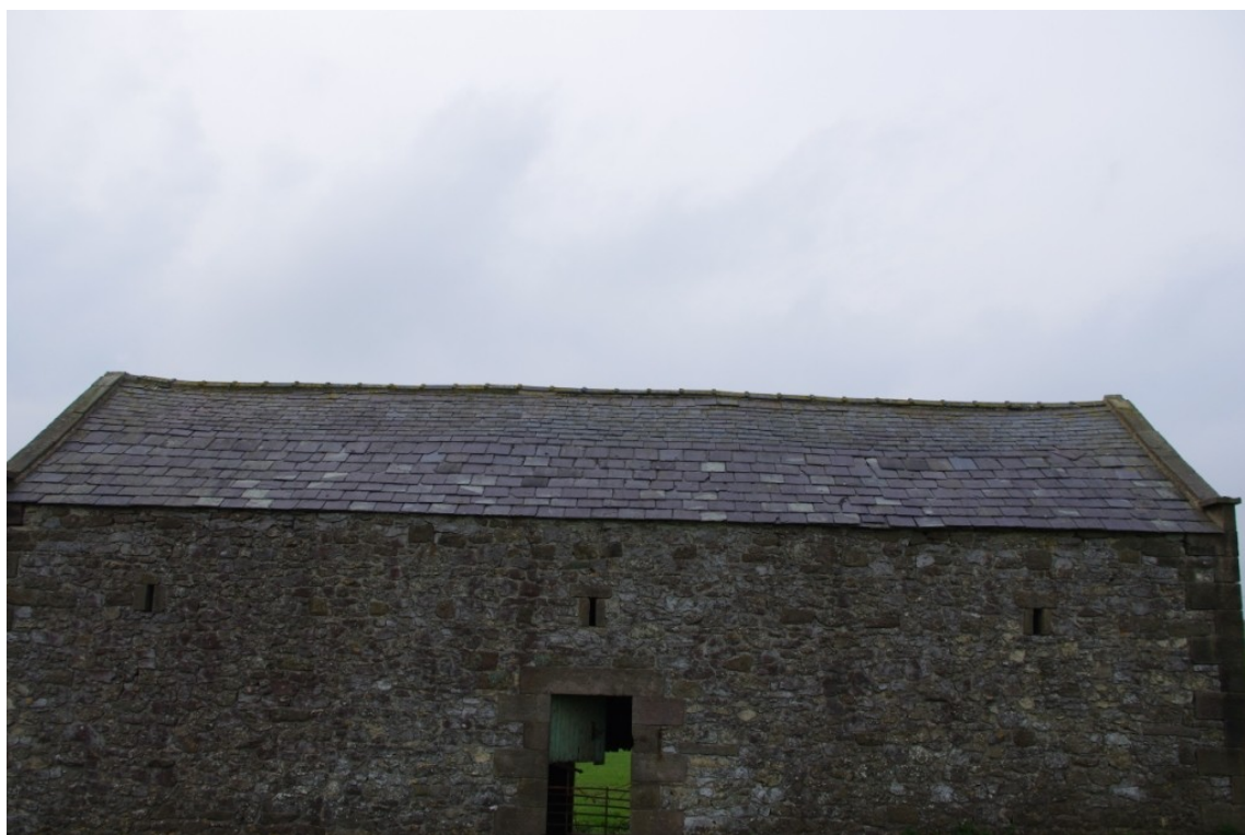
Figure 12 Two Phases of Roof & Graduating Slates on North Facing Roof.
