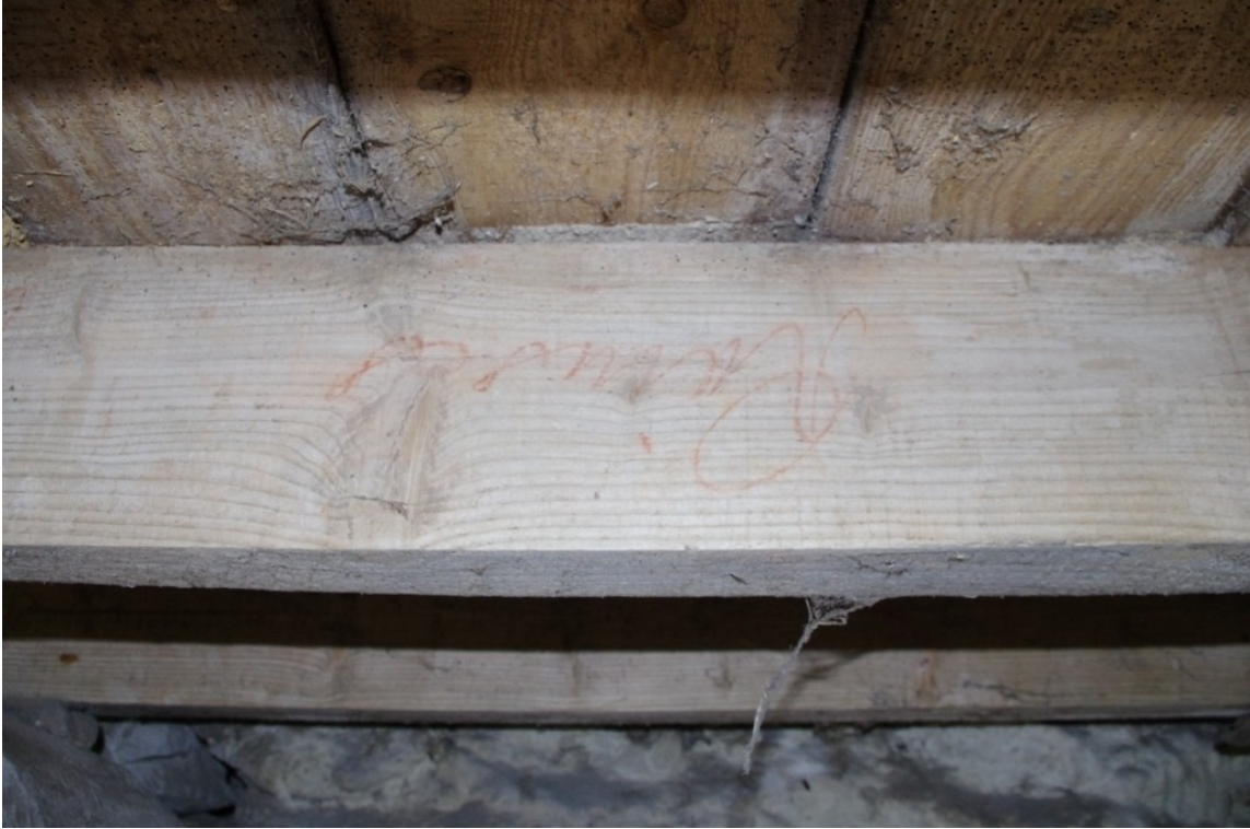
Figure 16 (3) 19th Century Graffiti on Joists.
