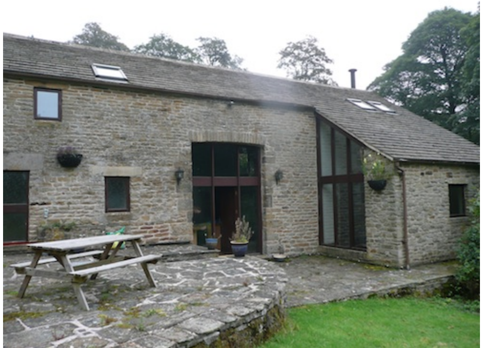
Fig.4 South (front) elevation of the original 17 th century barn with its former tall & wide single-entry cart entrance and later forward lean-to (possible former wheel or engine house or cornhole ?). The former door and window opening to the far left hand side most probably served a stable
