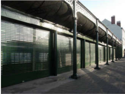
Doncaster Woolmarket – Repairs & alterations
